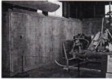
The new paneling and sloped cap are going up in Hangar 604.
